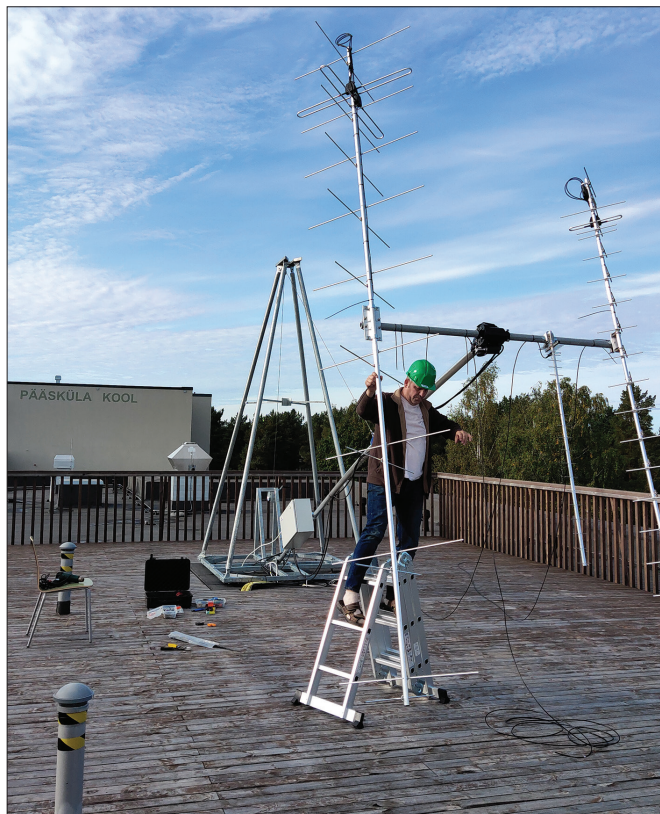
ES1TN SAT-side antennide paigaldamine
